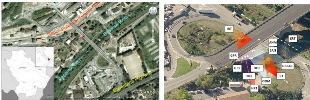
Fig. 1. (left) Location of Musmeci bridge - aerial view; (right) Locations of sensors on the Musmeci Bridge - upper view.
