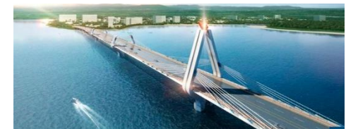
Tanzania New Selander Bridge
