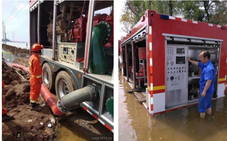
Figure 5: Shandong Shouguang drainage rescue
