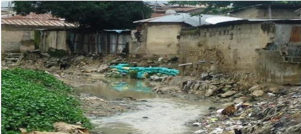
Plate I: Building on Flood Plane
