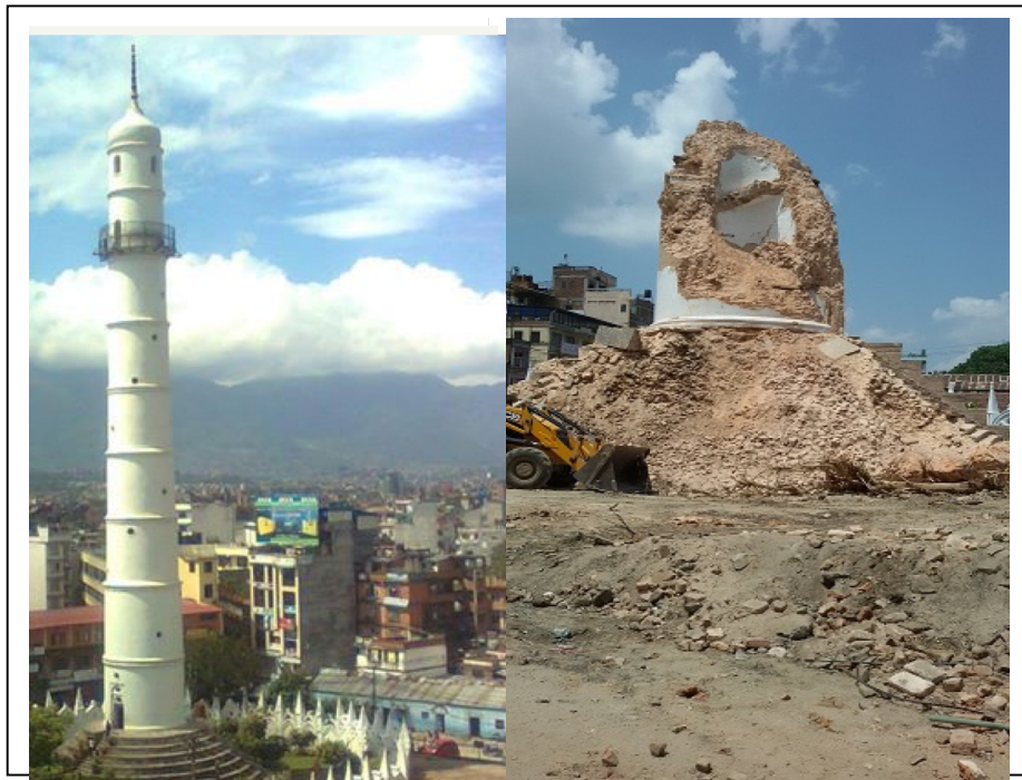
Picture 2: Dharahara (the view tower)—before the earthquake (left) & after the earthquake (right)
