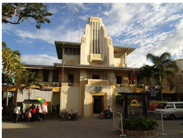
Figure 3 Calumpit Municipal Hall
