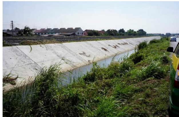
Figure 8 Railway acting as flood dyke near Ayutthaya
