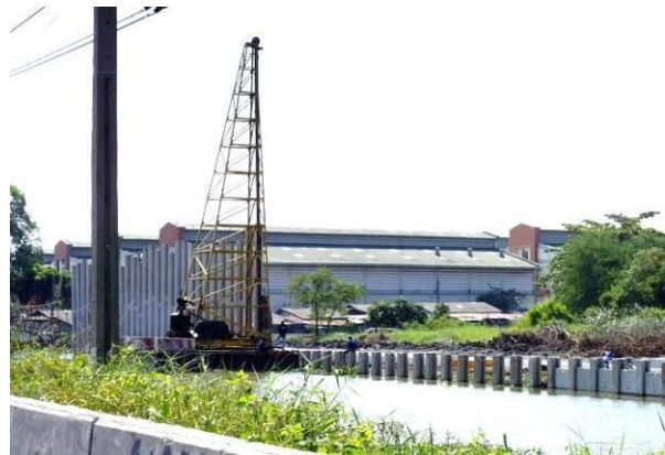
Figure 10 King's dyke upgrading eastern Bangkok (on-going work)
