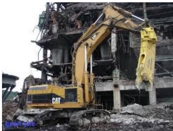
Figure 1. Backhoe with shear attachment
