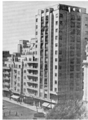
Figure 3. Carlton building in Bucharest, collapsed during 1940 earthquake
