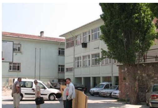
Figure 3. A vulnerable structure
