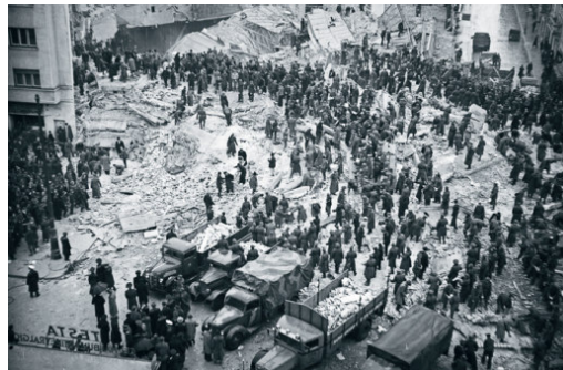
Fig. 2 Carlton Block site during debris removal (Photo Iosif Bergman, 1940)
