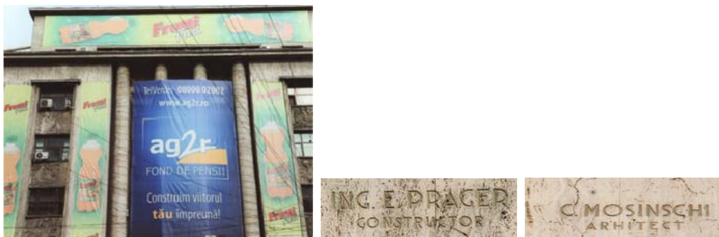
Figure 11. Façade of an historical building
