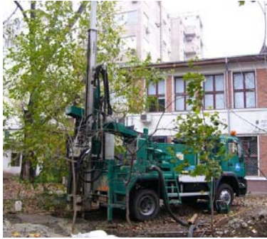
Figure 3. Drilling equipment on truck
