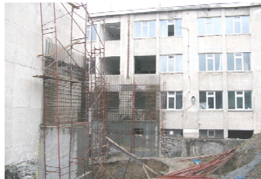
Figure 7. Construction of exterior concrete walls for a school retrofit
