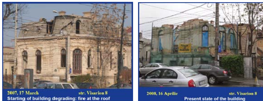
Figure 8. Bucharest heritage building in the city center intentionally prepared for demolition
