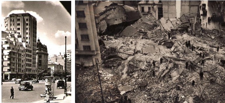
Fig. 1 Carlton Block before collapse (left) and immediately after collapse (right) (Photo: postcard and Ministry of Propaganda files, 1940)
