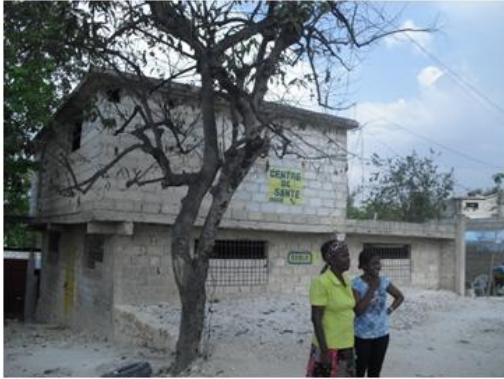
Figure 4. Overhanging Upper Floor
