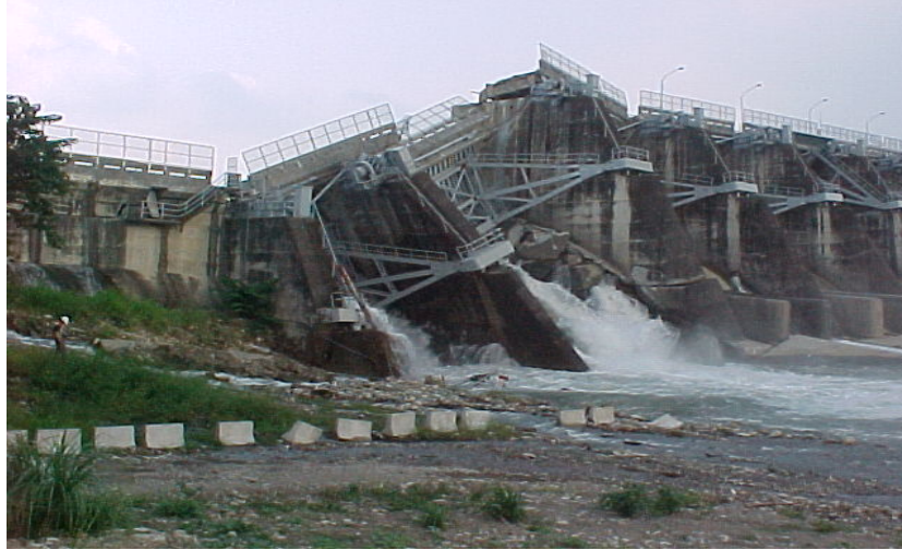
Figure 1. Taiwan Shih-Kang dam accident in a view (Dams4, 1999)
