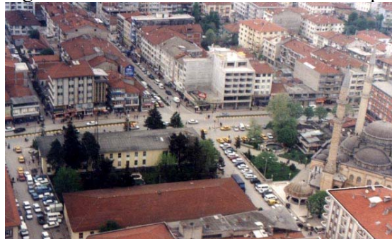
Figure 2 The Duzce City Center Before the Disaster
