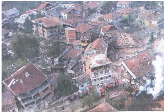
Figure 3 Duzce City Center after the Earthquake
