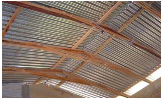
Fig 8: Completed roof
