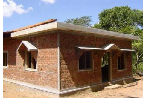
Fig 13: Completed flat concrete roof and sunsheds
