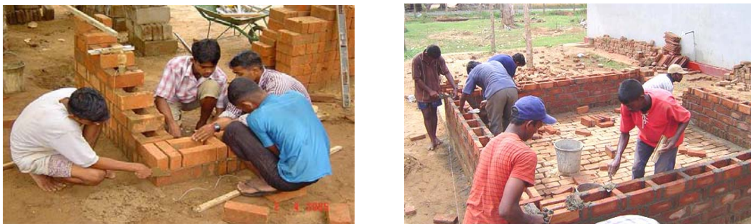
Fig 5: Wall construction in progress
