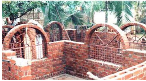
Fig 6: Arch preparation
