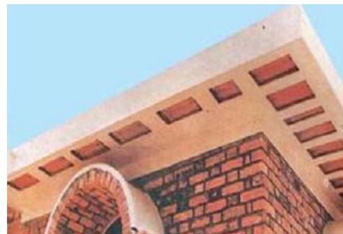
Fig 11: Completed filler slab and sunshade
