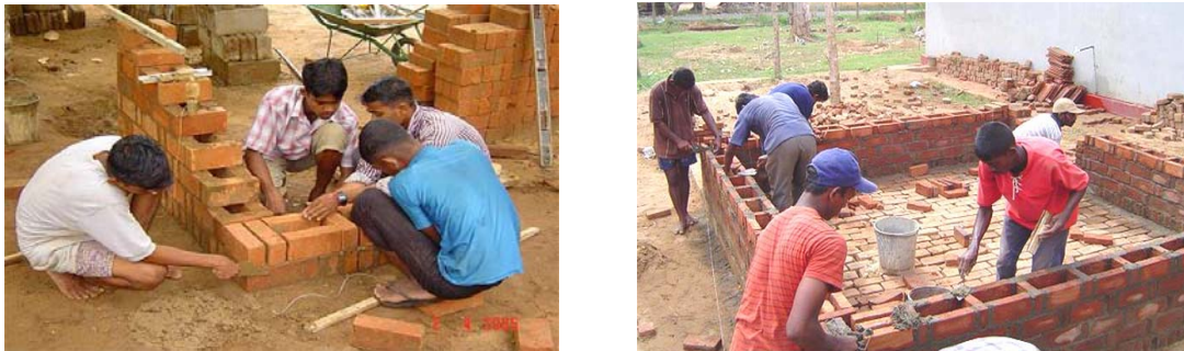
Fig 5: Wall construction in progress
