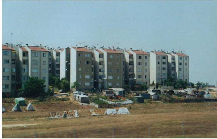
Fig. 8: User-built shelters near damaged apartment buildings in Turkey
