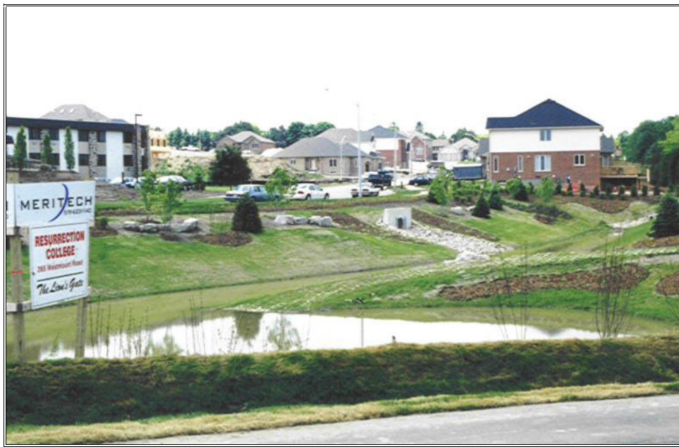
Figure 5: A Local Constructed Storm Water Detention Pond
