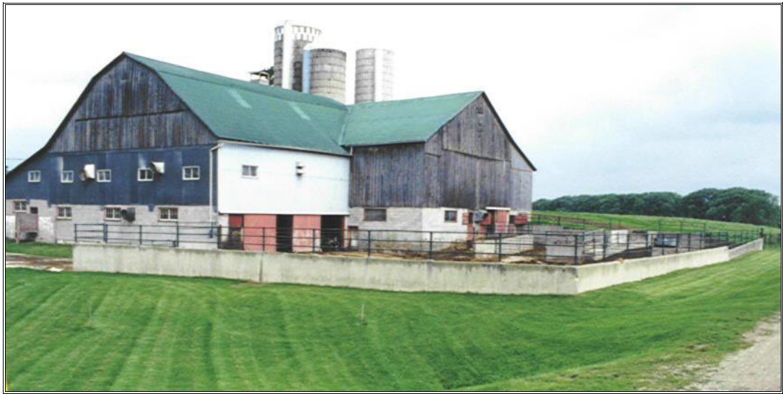
Figure 7: A Family Farm With Concrete Animal Waste Management Facilities
