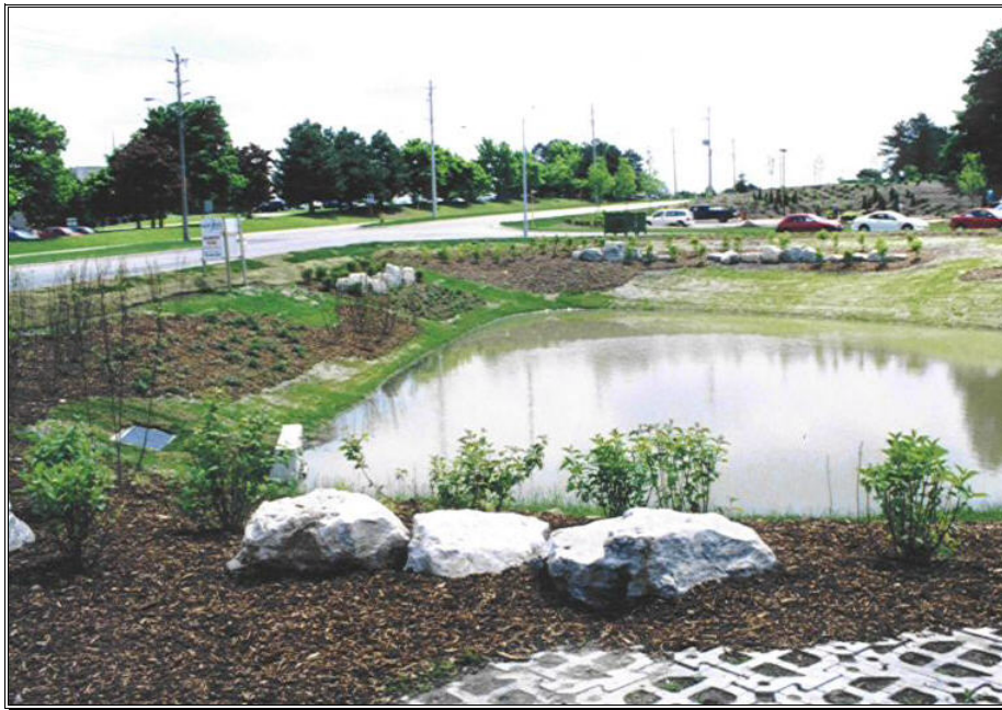
Figure 6: Constructed Storm Water Detention Pond and Discharge
