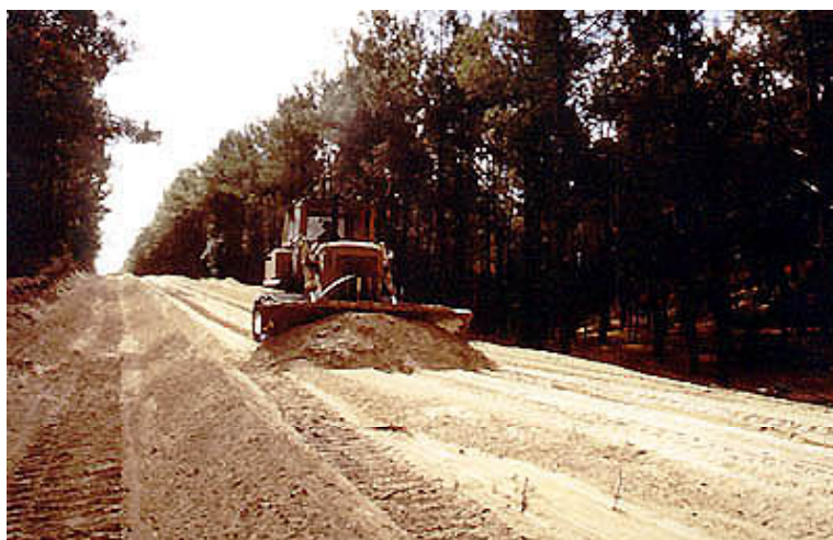
Figure 5. More spacious firelines or safety areas may be produced using bulldozers
